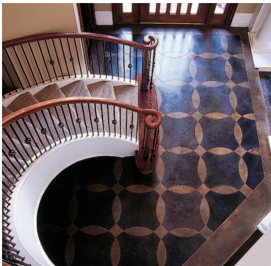
LEFT: An elegant floor is concrete stained and sealed with Kemiko products. BELOW: The “wave sink” by Stone Soup Concrete, ground and polished to expose aggregate and colored glass in the mix. BELOW LEFT: The “Biltmore” fireplace looks like Italian limestone [3000 from Sierra Designs].
