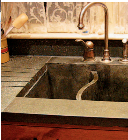
LEFT: An elegant floor is concrete stained and sealed with Kemiko products. BELOW: The “wave sink” by Stone Soup Concrete, ground and polished to expose aggregate and colored glass in the mix. BELOW LEFT: The “Biltmore” fireplace looks like Italian limestone [3000 from Sierra Designs].
